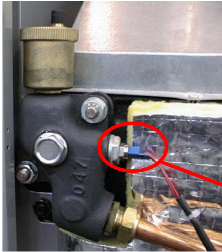
NTC probe positioned in the Heating Circuit
